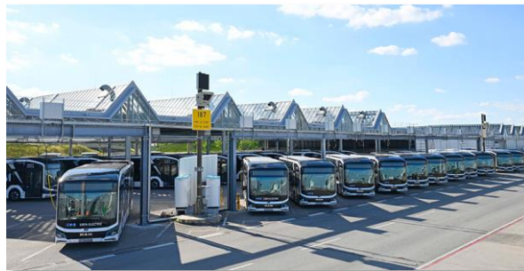
E-bus depot at Munich Airport | source: Munich Airport
